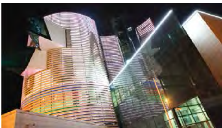
Socar Headquarters, Tbilisi - Georgia
