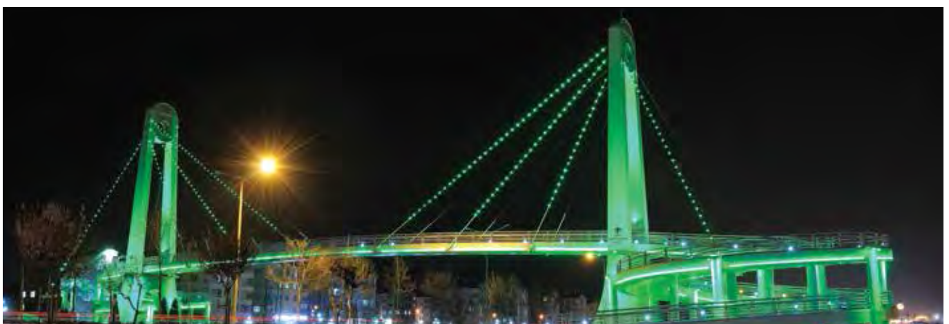
Elmalılı Hamdi Pedestrian Overpass, Konya - Turkey
